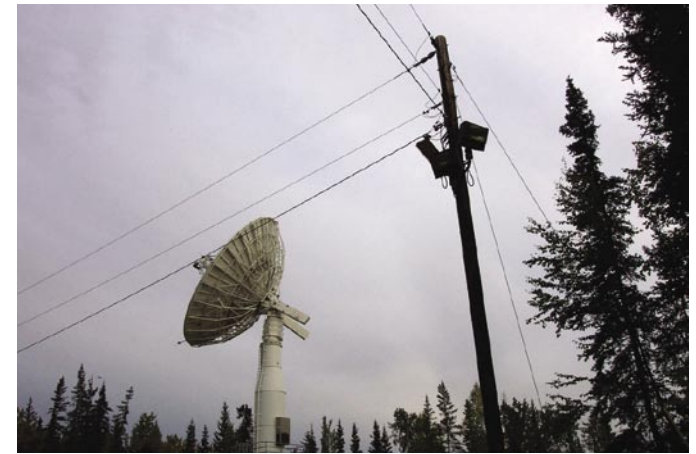
Power lines and Alaska SAR antenna in North Campus area.
