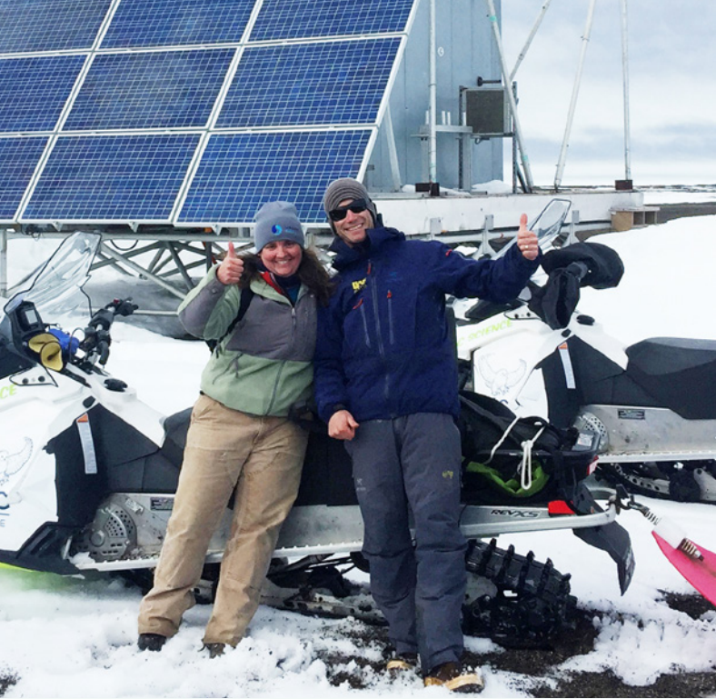
◀ Rachel Potter and Hank Statscewich conduct maintenance on a remote power system built at UAF for Point Barrow's HF radar. Photo by Qaiyaan Leavitt at UIC Science.
