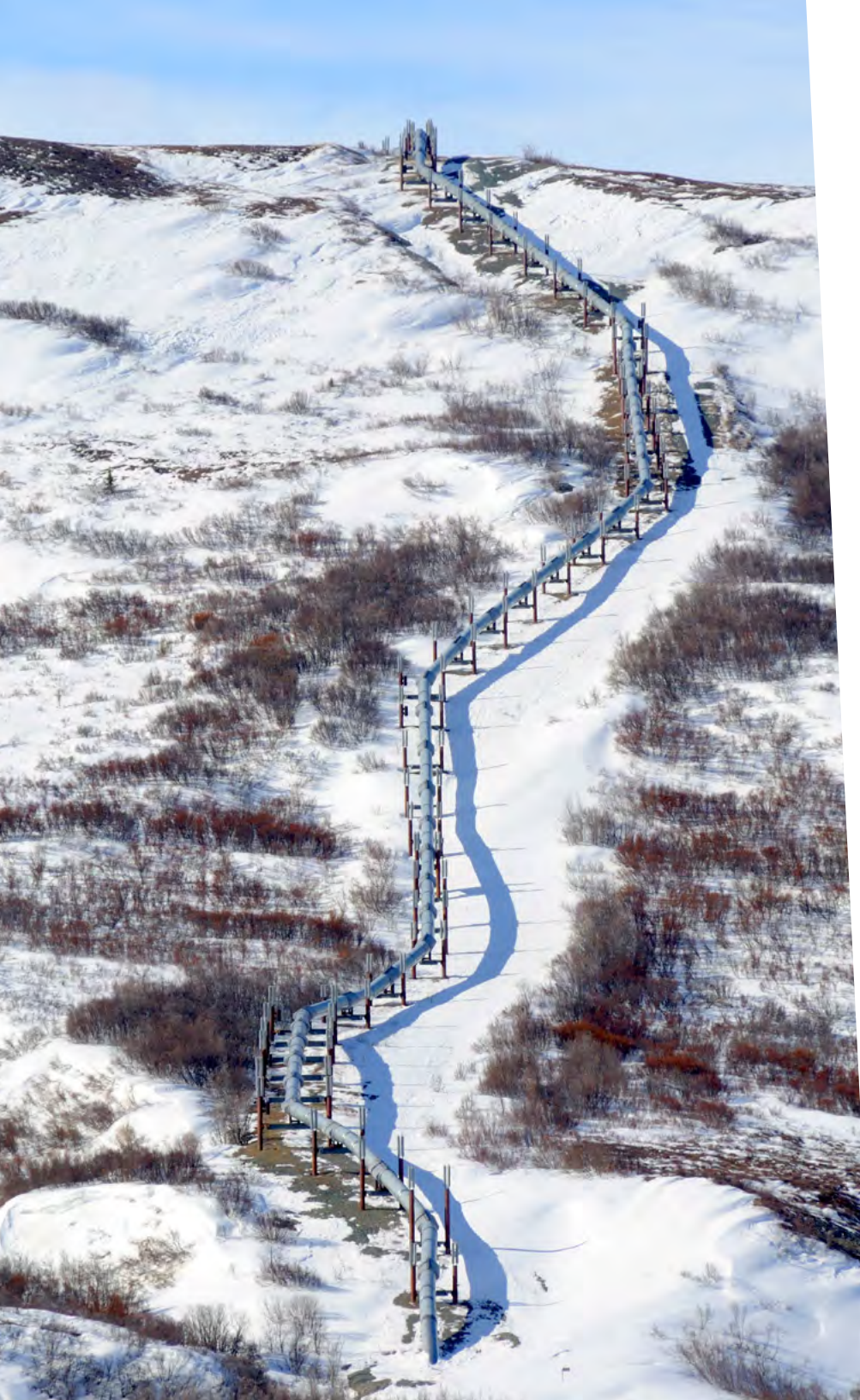
Trans-Alaska Oil Pipeline
