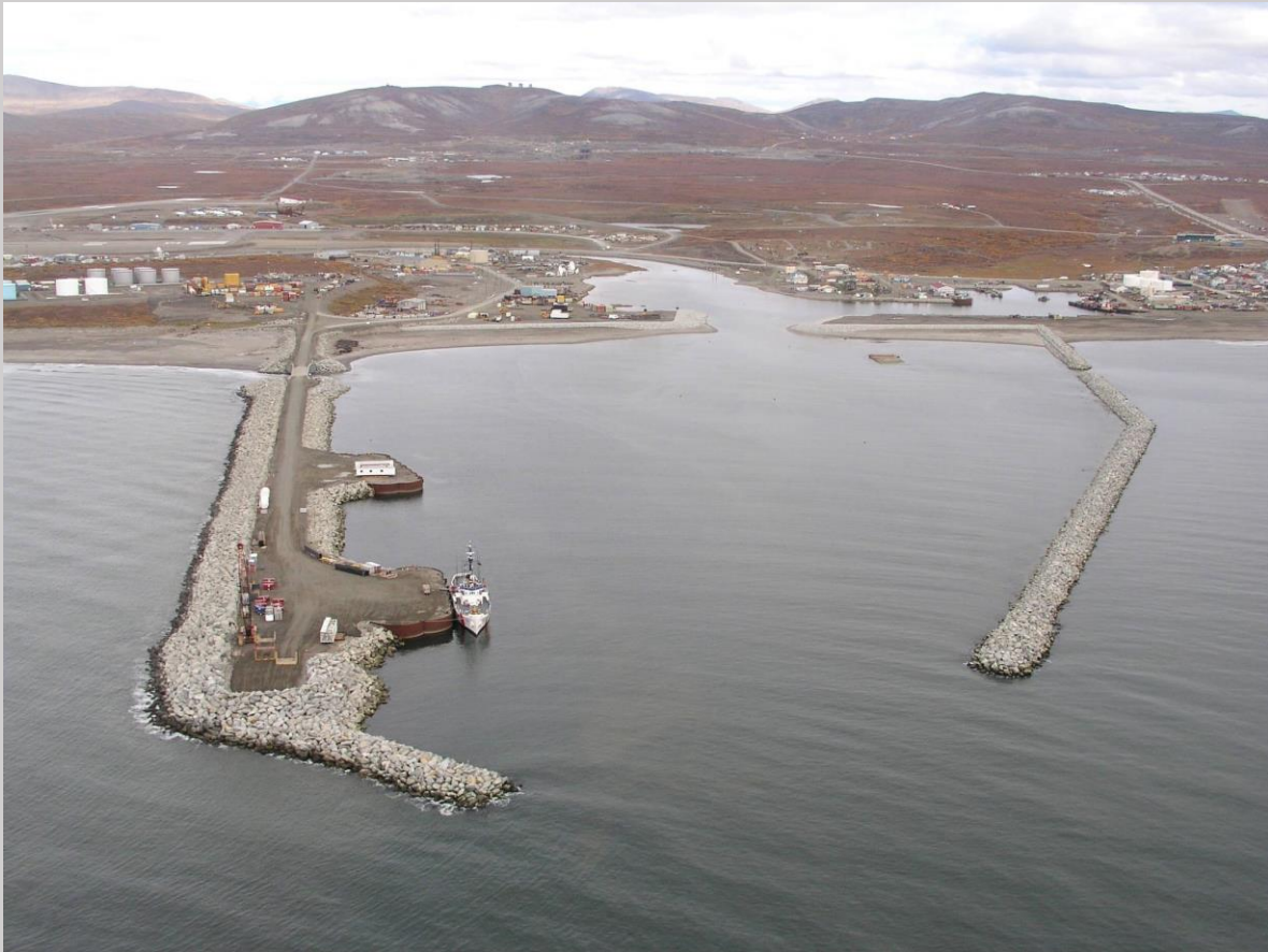
Figure 5. Existing infrastructure of the Nome port shown above. Photo courtesy of the US Army Corps of Engineers. Source:
