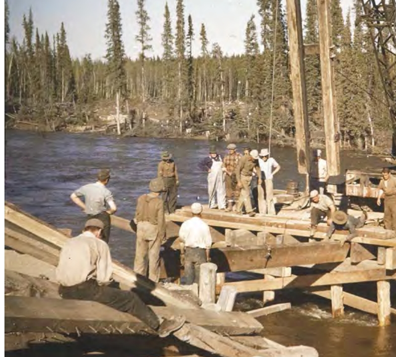
Highway workers repair an Alaska Highway bridge across a river south of Whitehorse, in Canada’s Yukon, in May 1948. High water that spring washed out parts of the road and its bridges. Dave Klein and a friend had to wait here briefly while driving his Model A back to the Lower 48.
